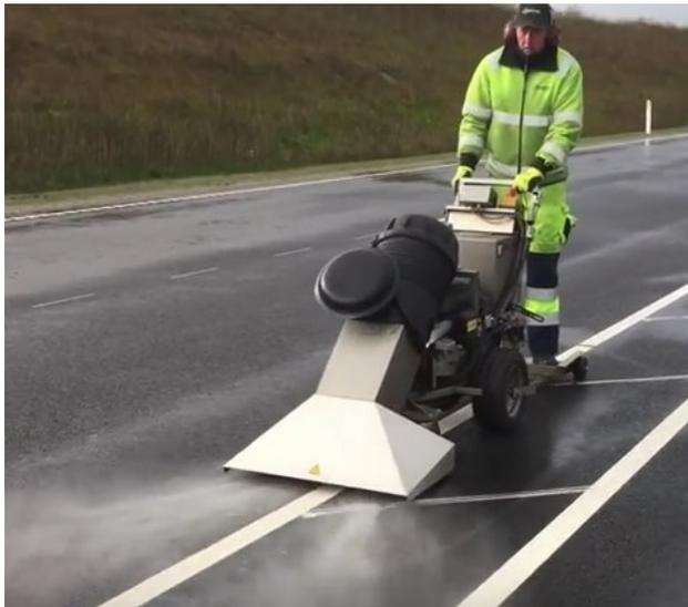
The fine alternative to heavy and hazardous LPG gas and diesel compressor systems, for drying out wet roads. Water, moist, traffic dirt, or the by sunlight worn-out top surface will disappear and so secure best adhesion for any new roadmarking or surface treatment.
